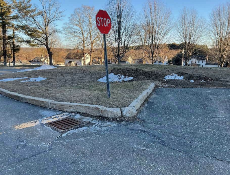
Existing catch basin that captures stormwater from south parking lot, facing south.
