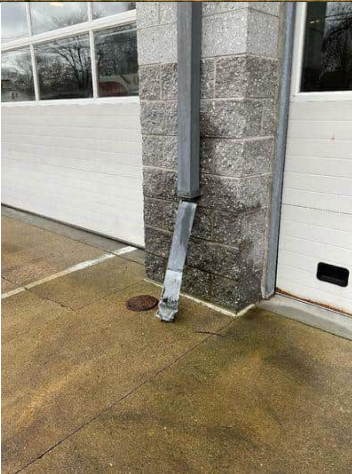
Disconnected downspout along fire department vehicle bay.
