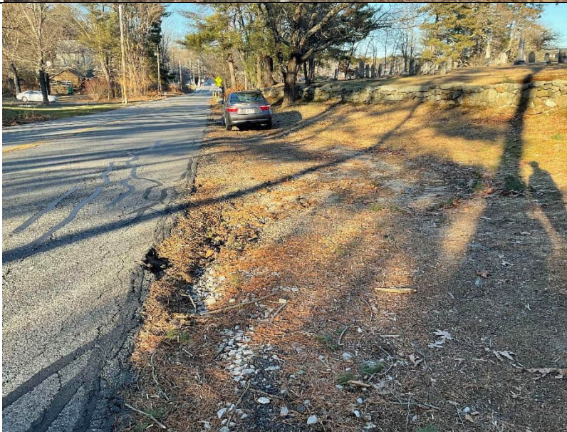
Existing channelized erosion along School St, facing north.
