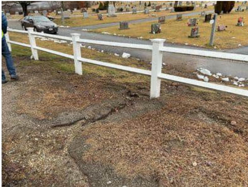
Channelized erosion entering site along North Main Street, with deposited sediment visible in background.
