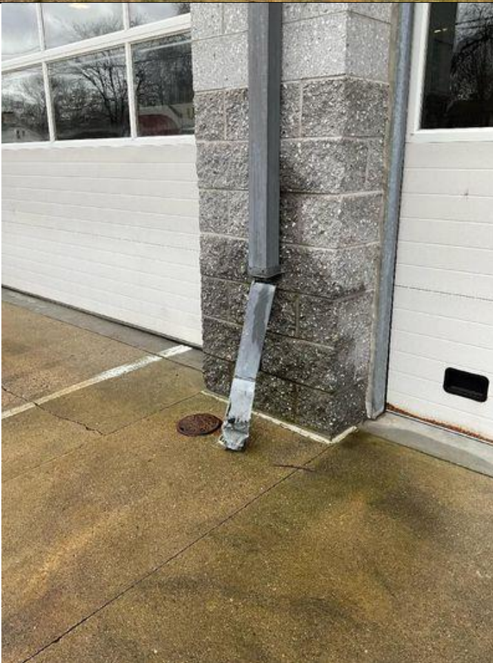
Disconnected downspout along fire department vehicle bay.
