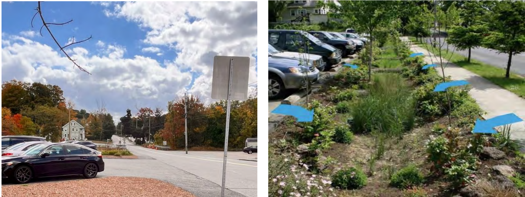
Figure 17 - Photo - Left: Existing town parking lot on Grove Street. Right: Parking lot runoff directed into a bioswale*
