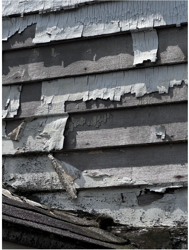
Peeling paint above the side entrance roof
