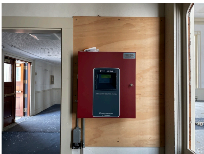
Fire alarm panel at front entrance
