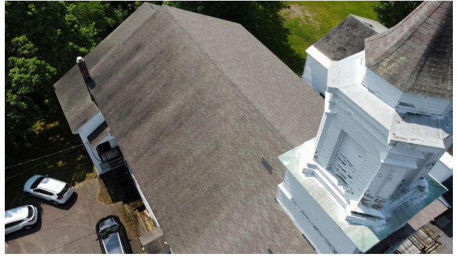
Left view of asphalt roof with missing shingles.
