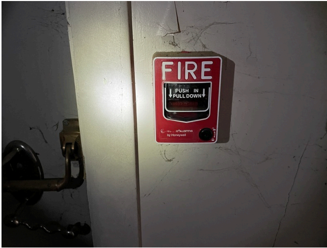
Example of a pull station
