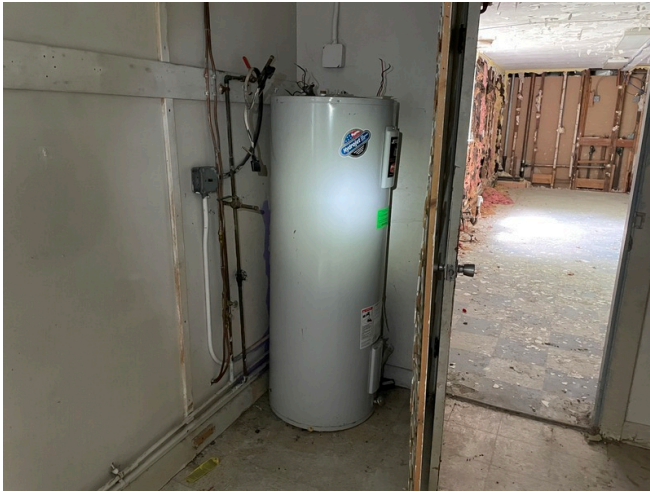
Electric water heater at left rear basement.
