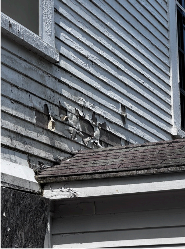
Roof over the side entrance door does not appear to be properly flashed and has resulted in water infiltration
