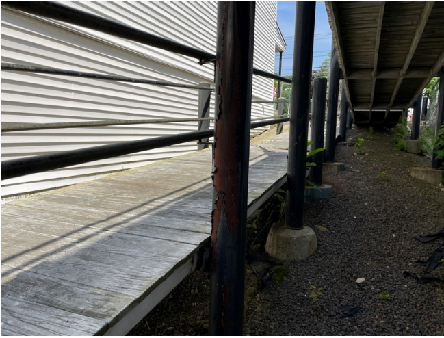
Bottom portion of the ramp. According to the laser scan, the slope is 1" per 12".
