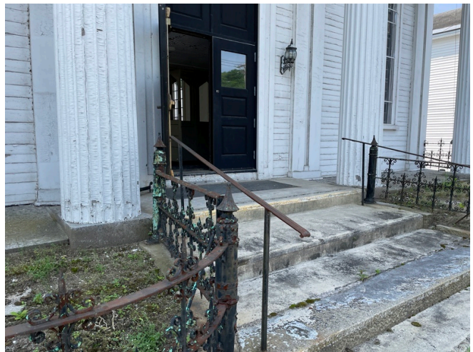
Front entrance. The concrete steps are in poor condition.
