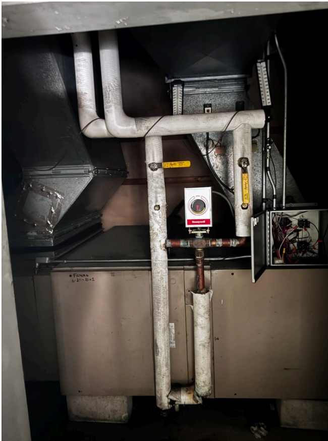
York Air Handler located at the left rear of the basement
