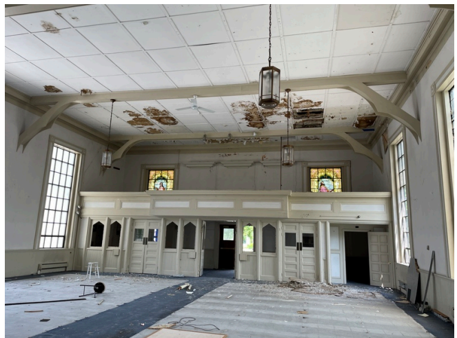
View looking toward the front of the building. Note the water staining on the ceiling.
