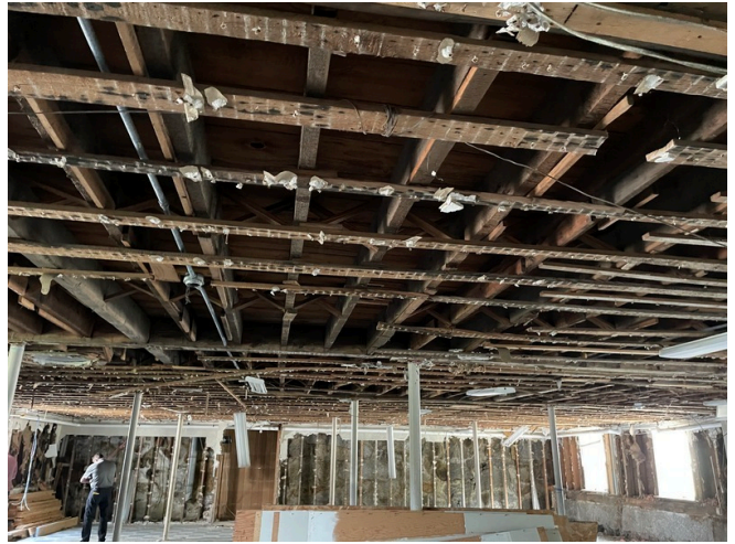
Basement with first floor framing exposed
