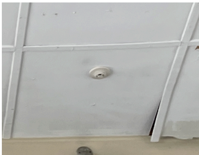
Example of a heat detector
