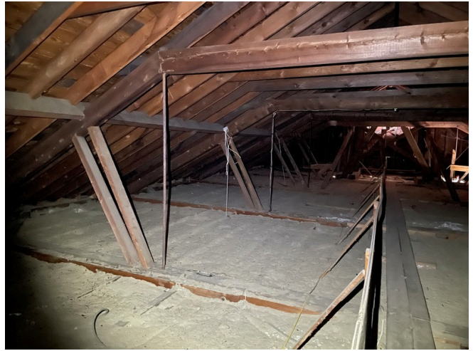
Exposed framing in the attic. Note the ceiling insulation
