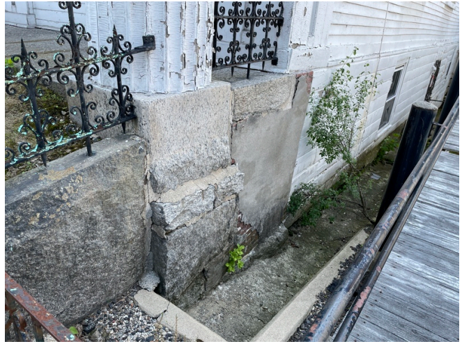
Right side of the building. Right front brick support wall is damaged
