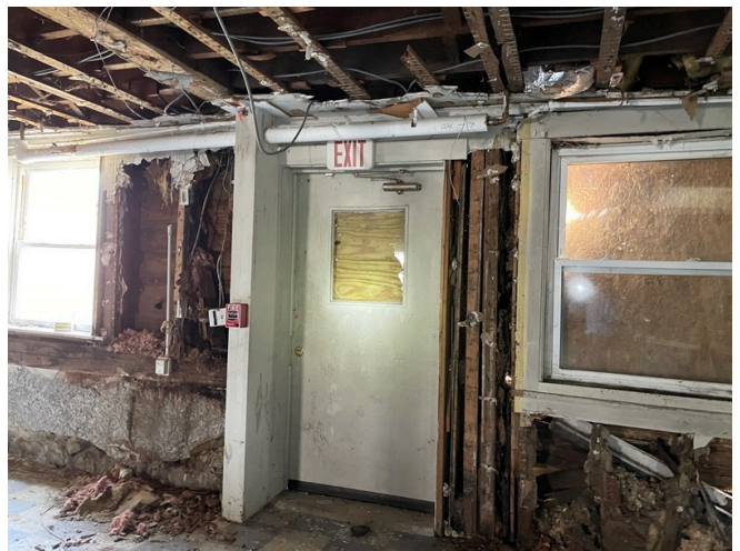
Left side wall that has been impacted by water infiltration
