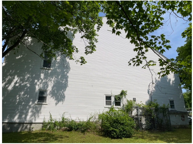
Rear of the church is covered in vinyl siding. Beneath the vinyl siding is shiplap up to the first level and wood clapboard above.
