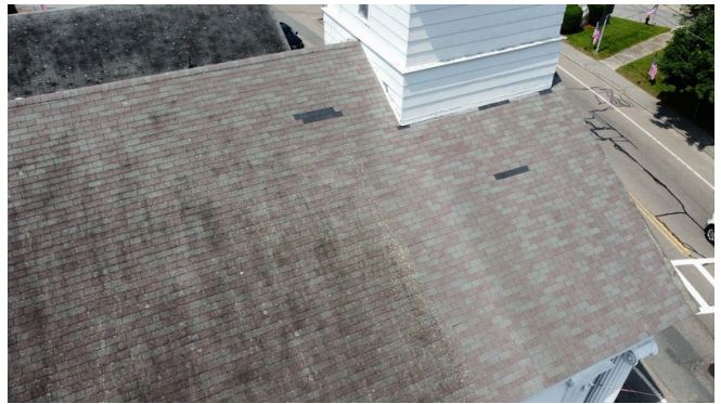
Close up of missing shingles and transition from steeple to asphalt roof. Visible staining on shingles
