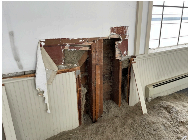
View of a support post in the walls.
