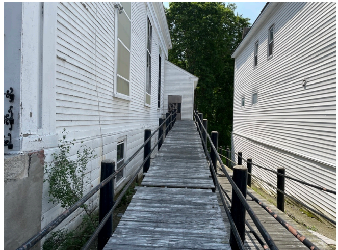
View of the ramp going up to the door. According to the laser scan, the slope is 1" per 12".
