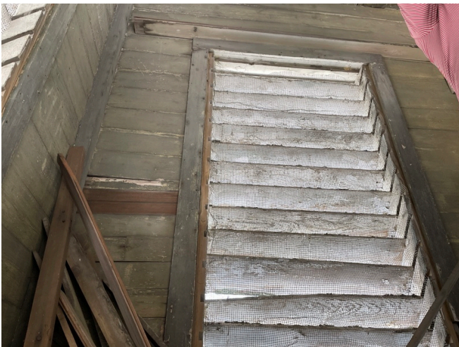
The top of the steeple was open to the elements through louvered openings
