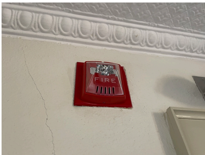
Example of an audible and strobe alarm
