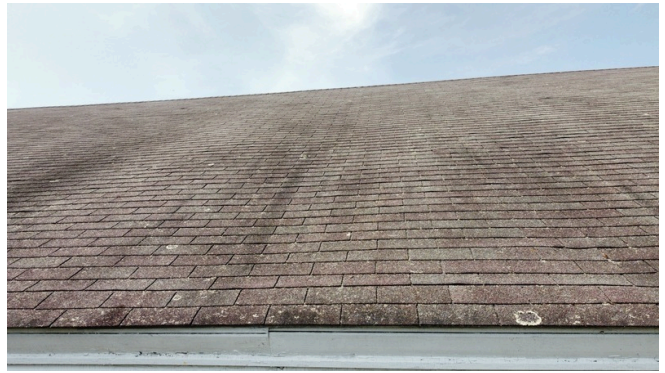
Visible staining and organic growth on asphalt shingles
