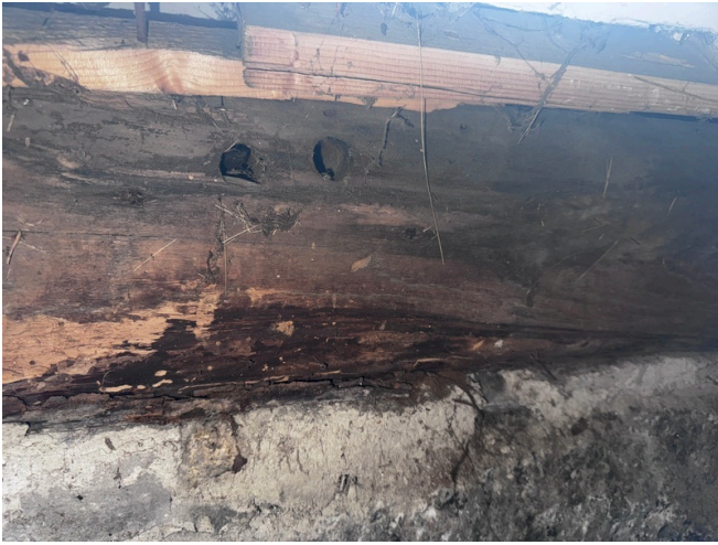
An example of the deteriorating sill plate/beam on the left wall.
