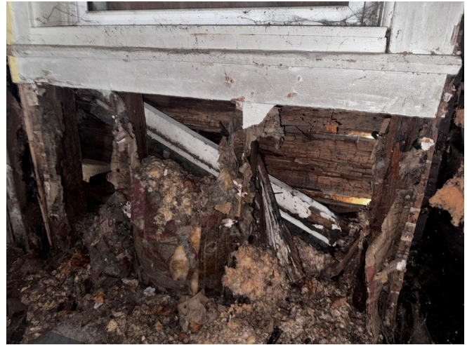
All studs, including king and jack studs under weindow is rotted. Exterior wall sheathing is rotted and daylight is observed.
