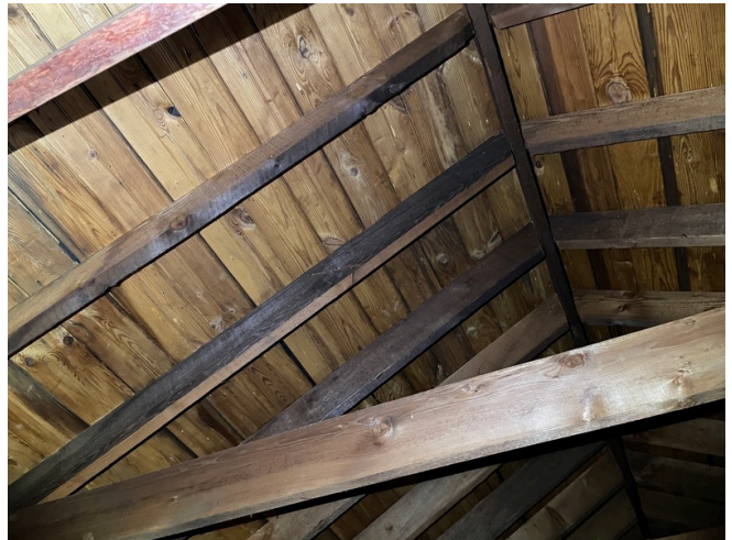
Rafters and roof sheathing
