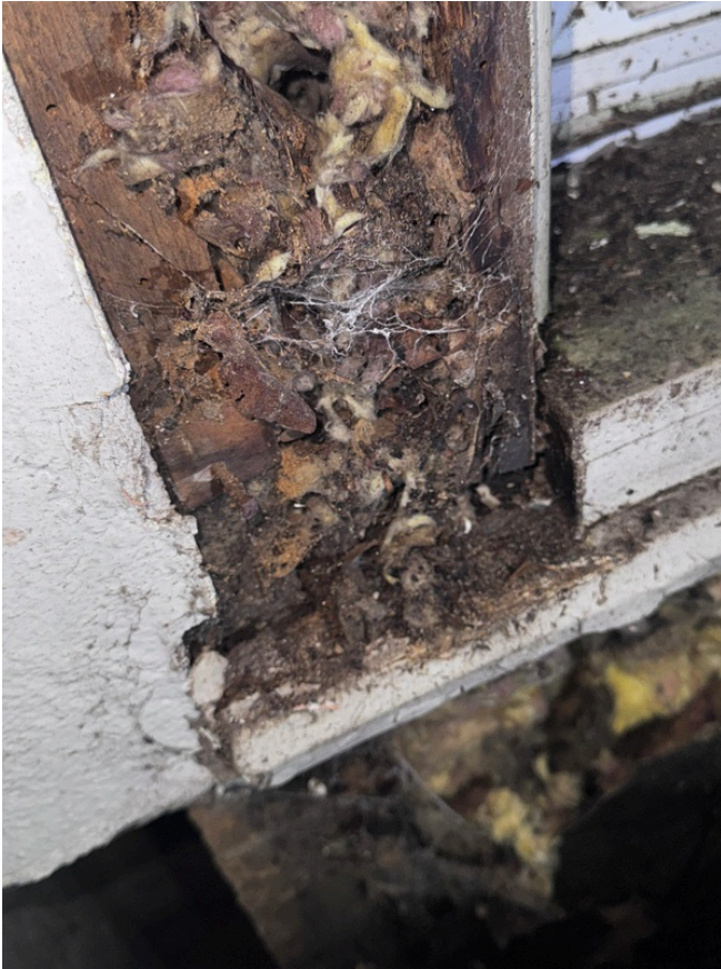
Exapmle of a window rough opening completely rotted.
