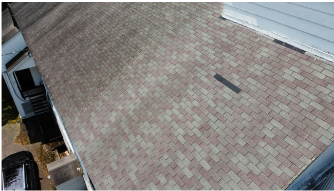
Close up of missing shingles and transition from steeple to asphalt roof
