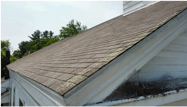
Organic growth on the asphalt shingles
