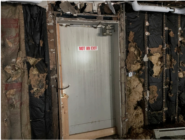
Right side wall around the door impacted by water infiltration
