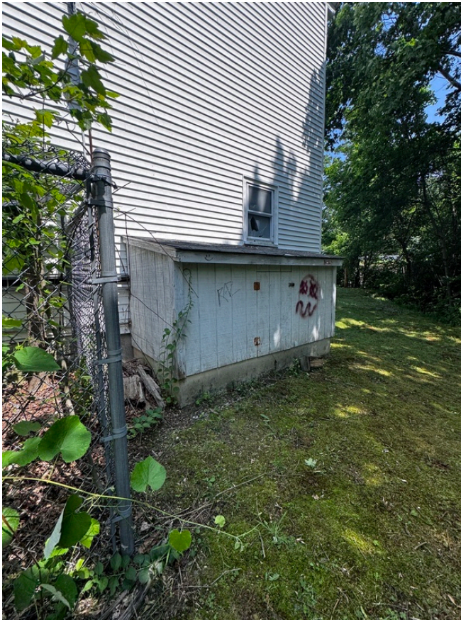
Oil tank enclosure
