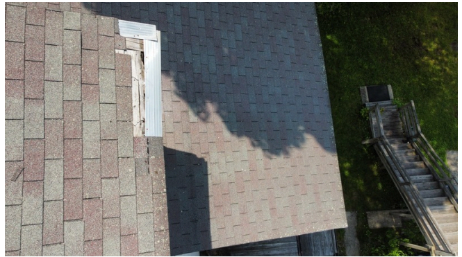
Missing shingles at rear right corner of main roof
