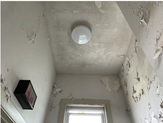
Example of peeling paint
