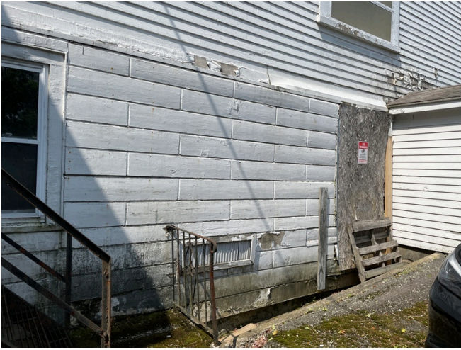
Siding in the area where there is water damage
