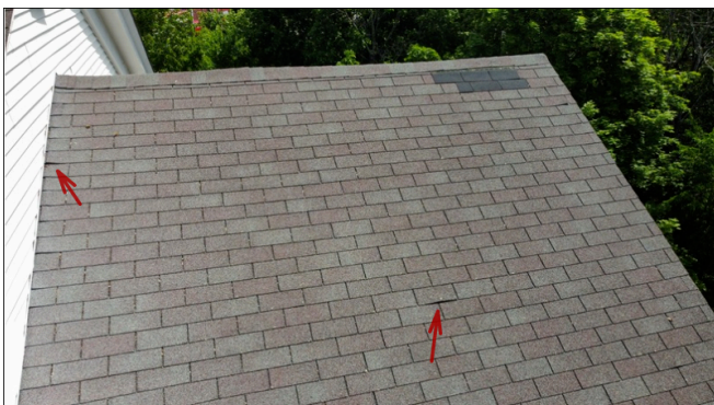
Rear small roof with lifted shingles
