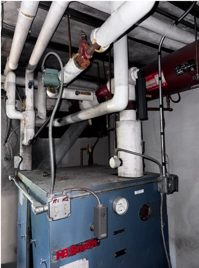
Oil fueled hot water boiler for heat
