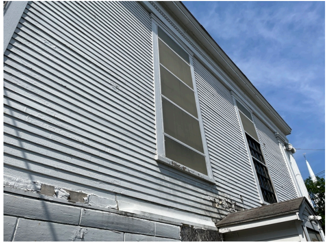
View of the siding. Note the peeling paint
