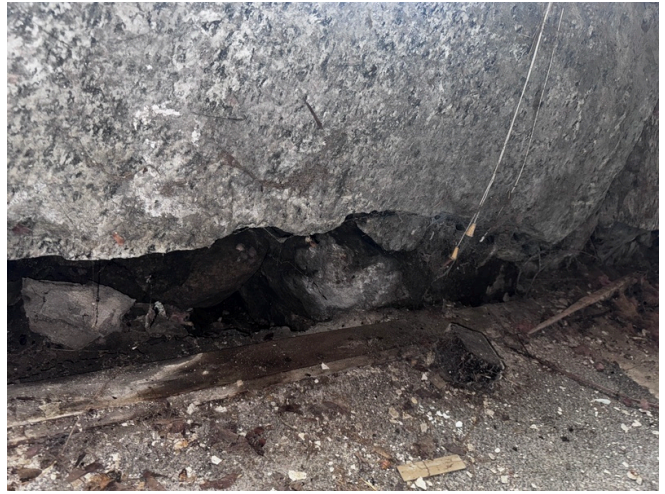
The base of the granite stone wall on the left foundation with missing stones.
