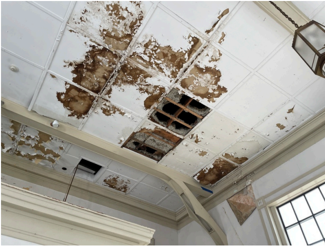
Water damage on the ceiling, located below the steeple.
