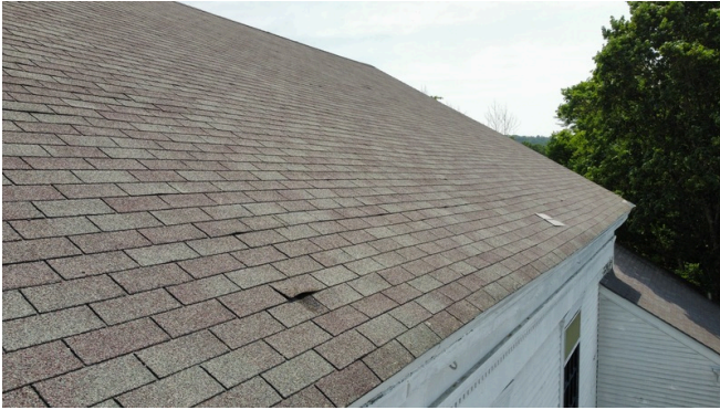
Right side of roof with raised and loose asphalt shingle
