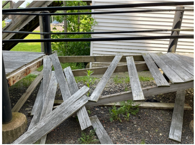
Damage to the ramp decking.
