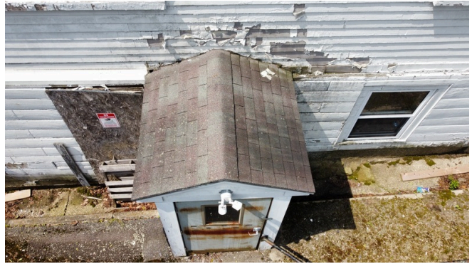
Stained small entrance roof with peeling paint on wood siding
