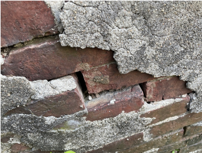
Brick in the right front support wall is displaced and mortar is degraded.
