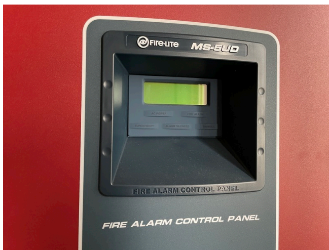
Fire alarm panel is not on
