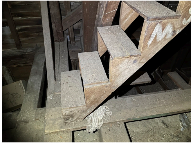
Stairs to the steeple. These were unstable and should be replaced
