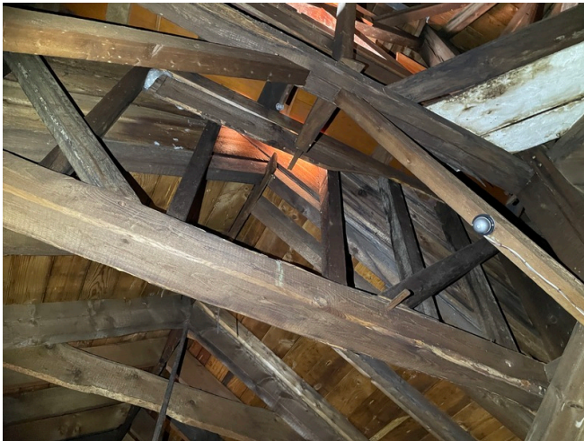
Wood and steel rod truss
