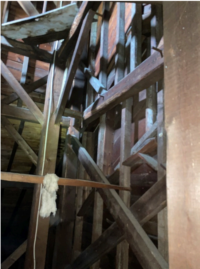
Post and beam framing of the steeple
