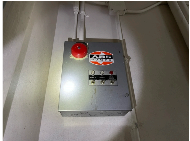
Sewage pump up controller
