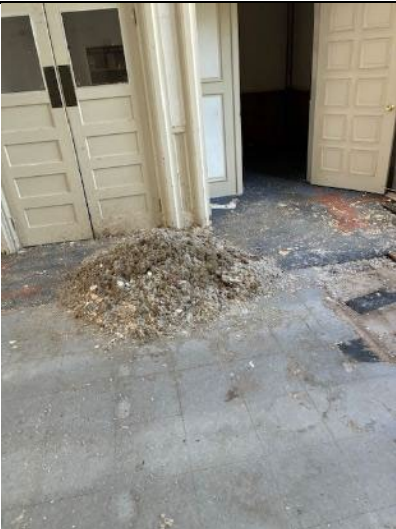
Overview of 1 st floor – asbestos containing tan 9" x 9" Floor tile extends beneath gray tile and carpeting
