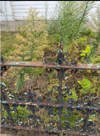
Lead-based black paint on metal railing
