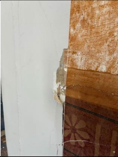
Lead-based red paint on plaster
