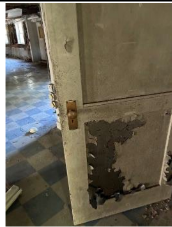
Lead-based white paint on metal door in basement
