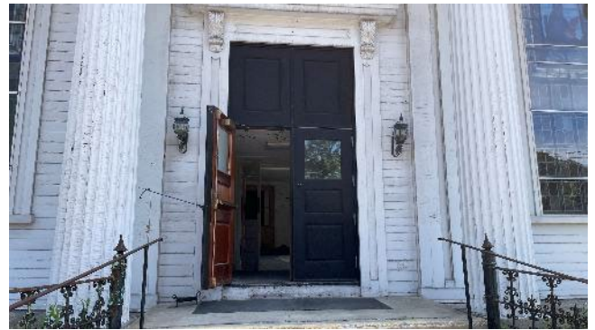
Lead-based paint on metal railings and front columns
