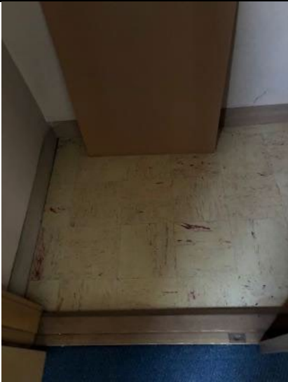
Asbestos containing tan 9" x 9" flooring in the first floor
