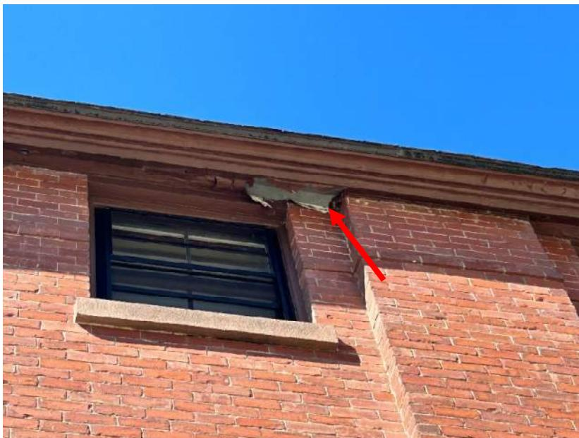
*Peeling / failed paint at eaves. Note that the roof in this area drains directly over the edge with no gutter.*
