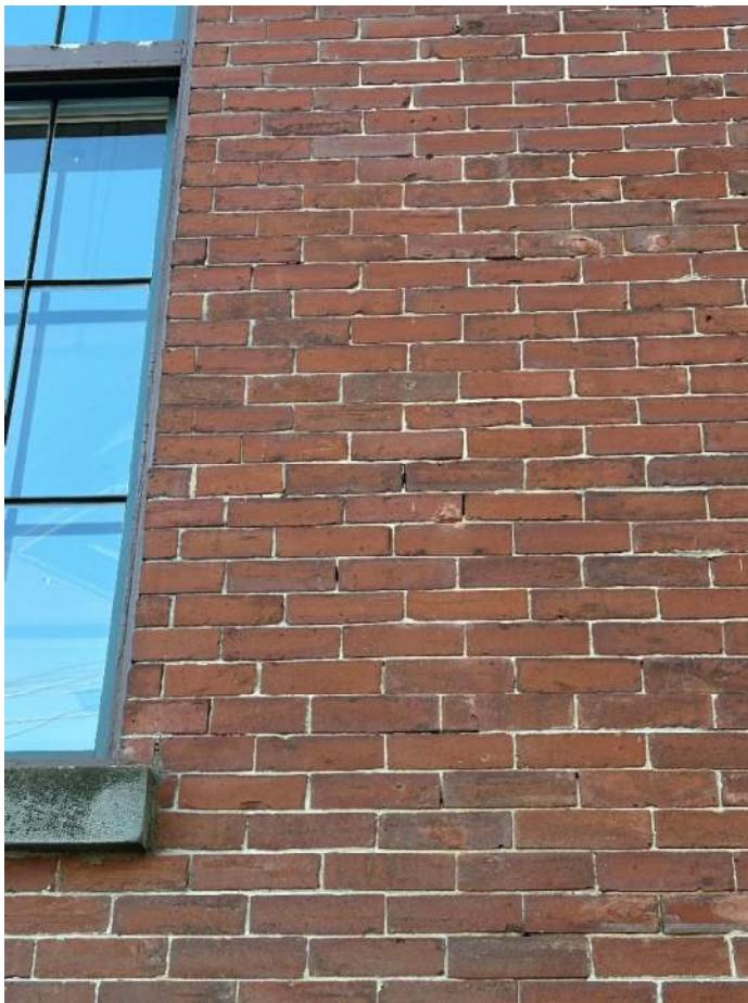
*Deteriorated mortar joints at North elevation.*
