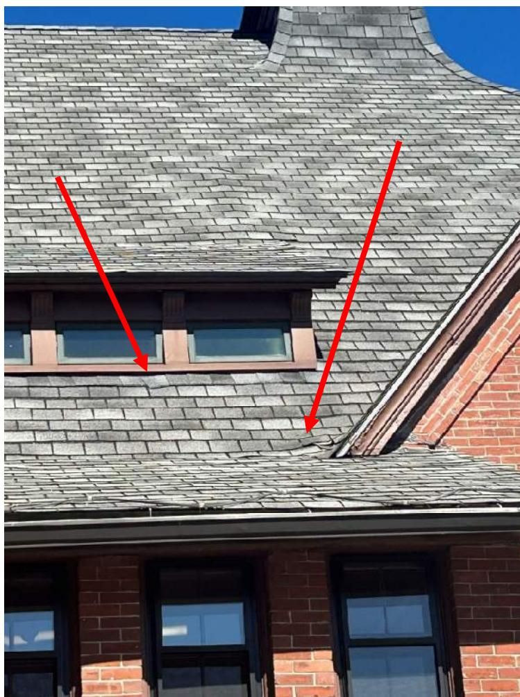
*South elevation – lifted shingles at bottom of a valley, and damaged shingles at a dormer rising wall.*
