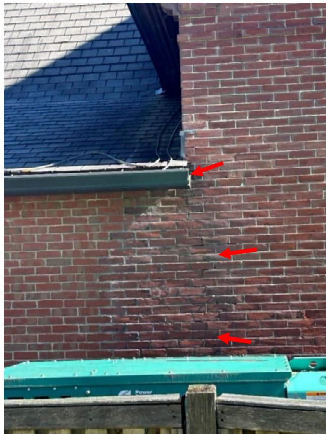
*Deteriorated and discolored brick below a gutter with no kickout flashing.*
