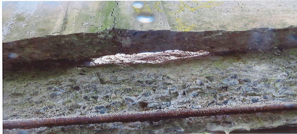
Photo 1: Hole found at the interface between the west railing base and top of deck.
