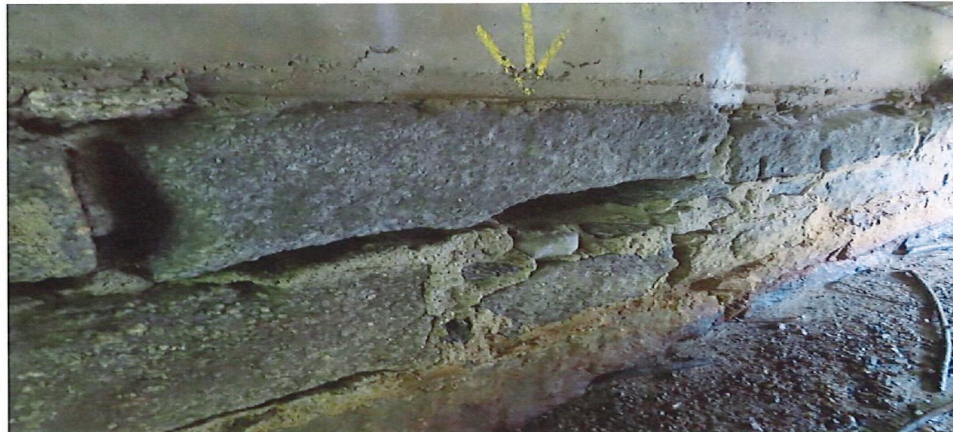
Photo 14: South breastwall void at midspan.
