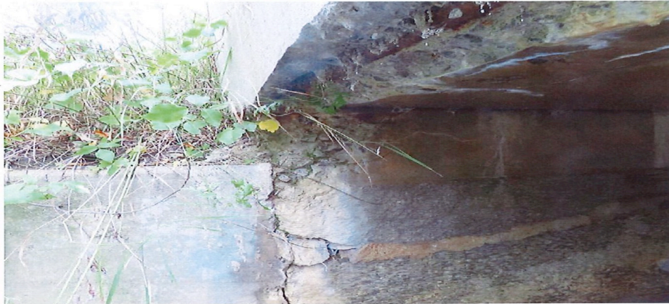
Photo 13: North breastwall scaling at the west end.
