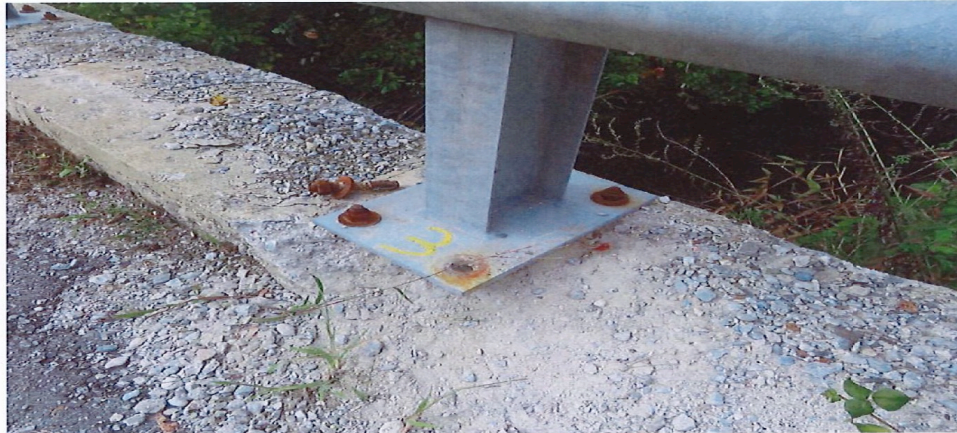
Photo 7: West railing, post #3 and heavy scaling.
