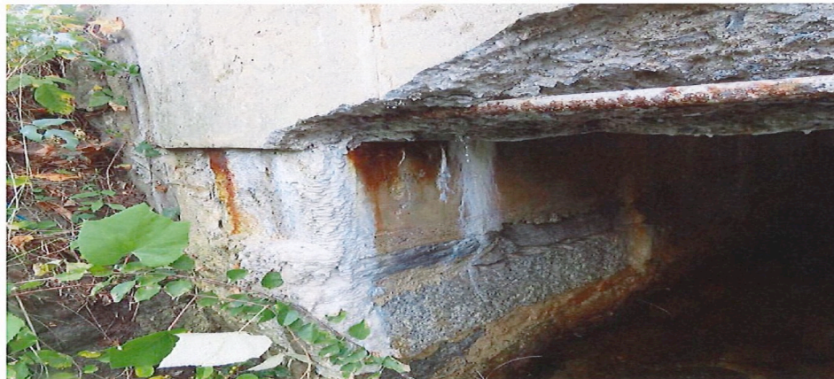
Photo 12: Southeast corner of breastwall efflorescence and rust staining.
