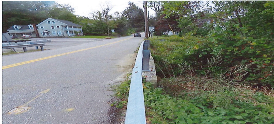
Photo 9: West railing tilting out towards the channel.
